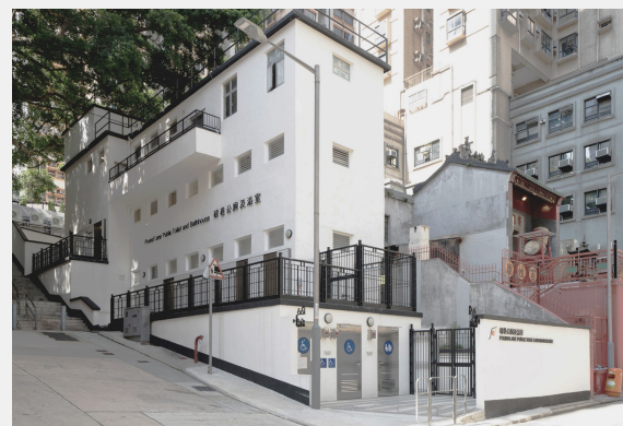
Figure 5. Pound Street Toilet after refurbishment, 2023
