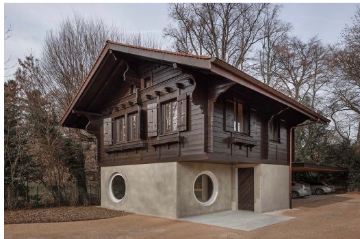
Mr Barrett's House by BUREAU
